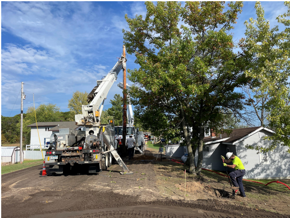
Photo #2: Relocating power pole away from causeway - Oct 2, 2023, 10:50 AM
