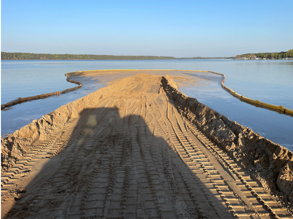
Photo #3: Beginning to build causeway for the inlet structure - Oct 2, 2023, 5:41 PM
