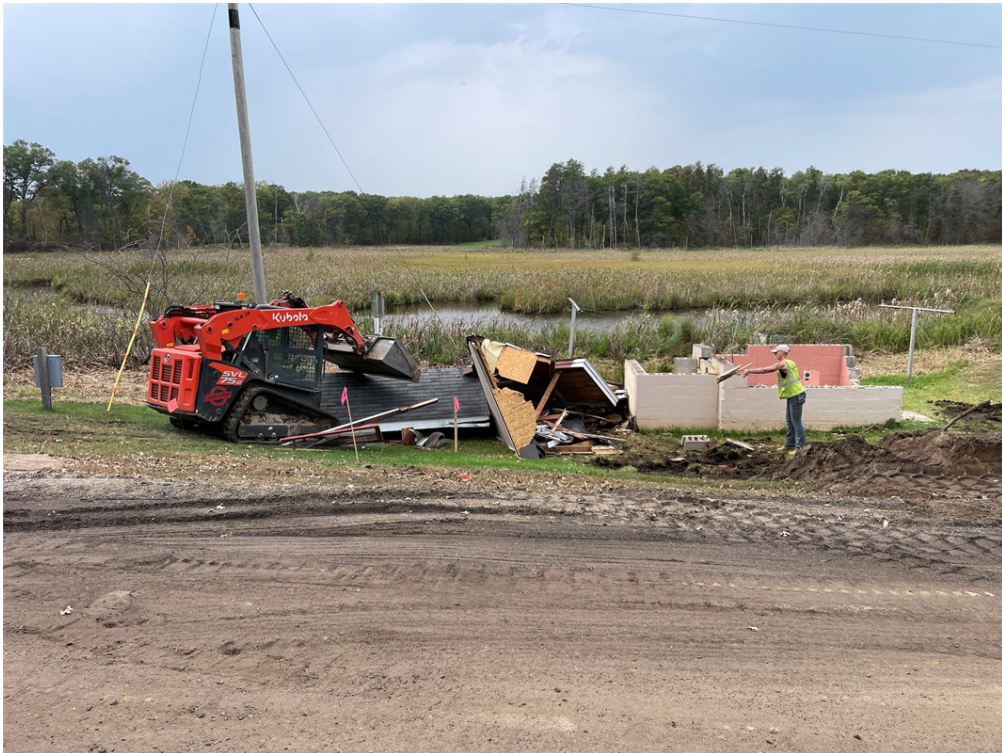
Photo #6: Remove fish cleaning house. - Oct 3, 2023 2:28 PM
