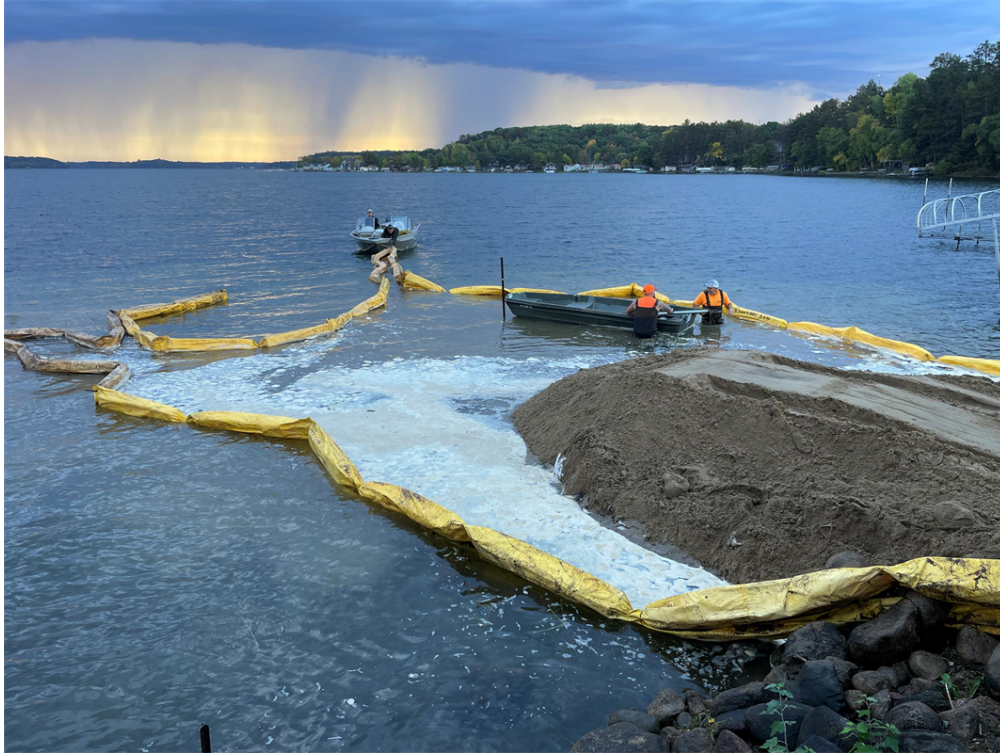
Photo #1: Installing floatation silt curtain around causeway - Oct 2, 2023, 8:33 AM
