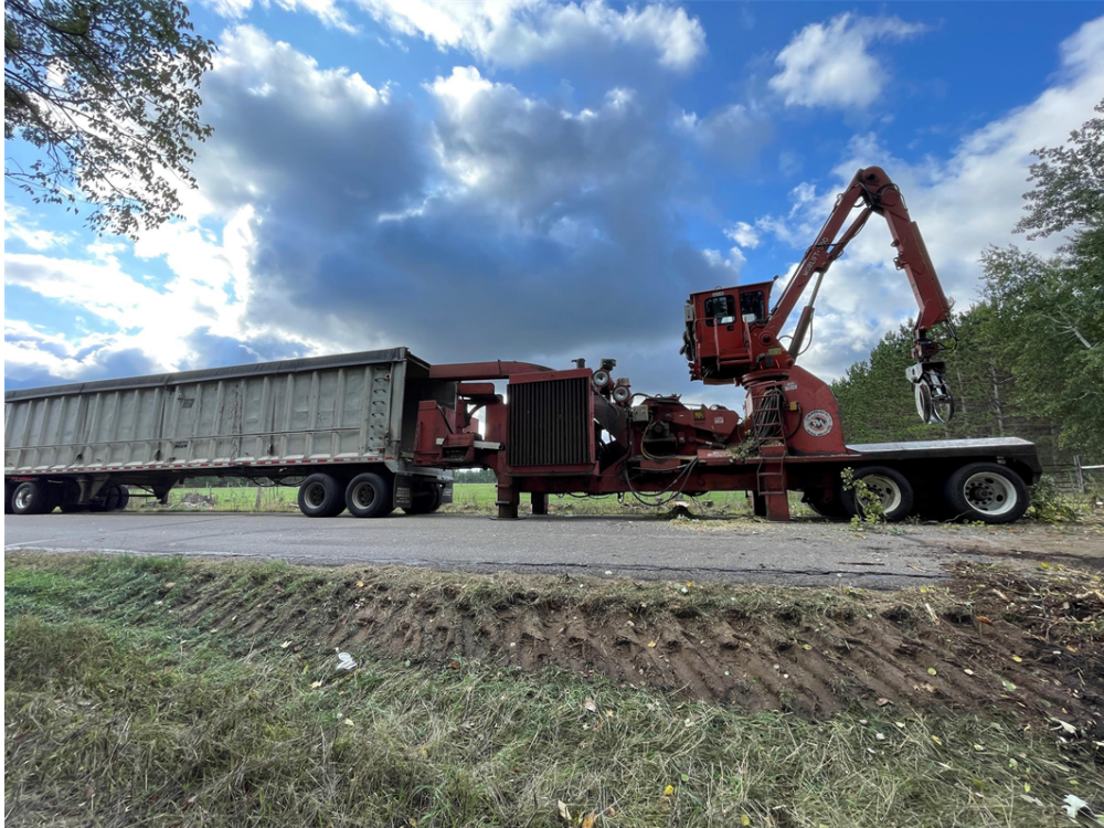
Photo #7: Clearing and grubbing with woodchipper - Oct 5, 2023, 2:49 PM
