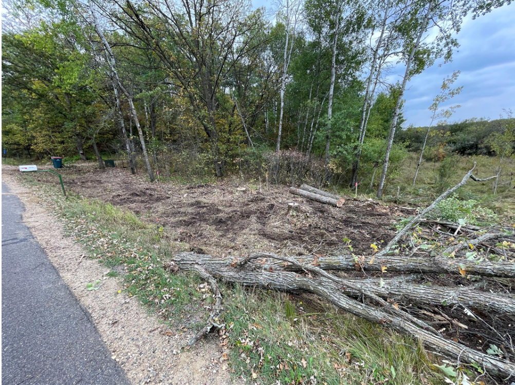
Photo #5: Clearing and grubbing on Pulaski Road - Oct 3, 2023, 2:10 PM
