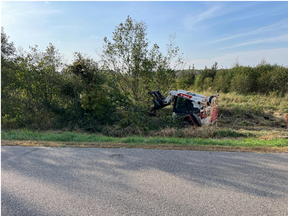
Photo #4: Beginning to clear and grub - Oct 3, 2023, 9:18 AM
